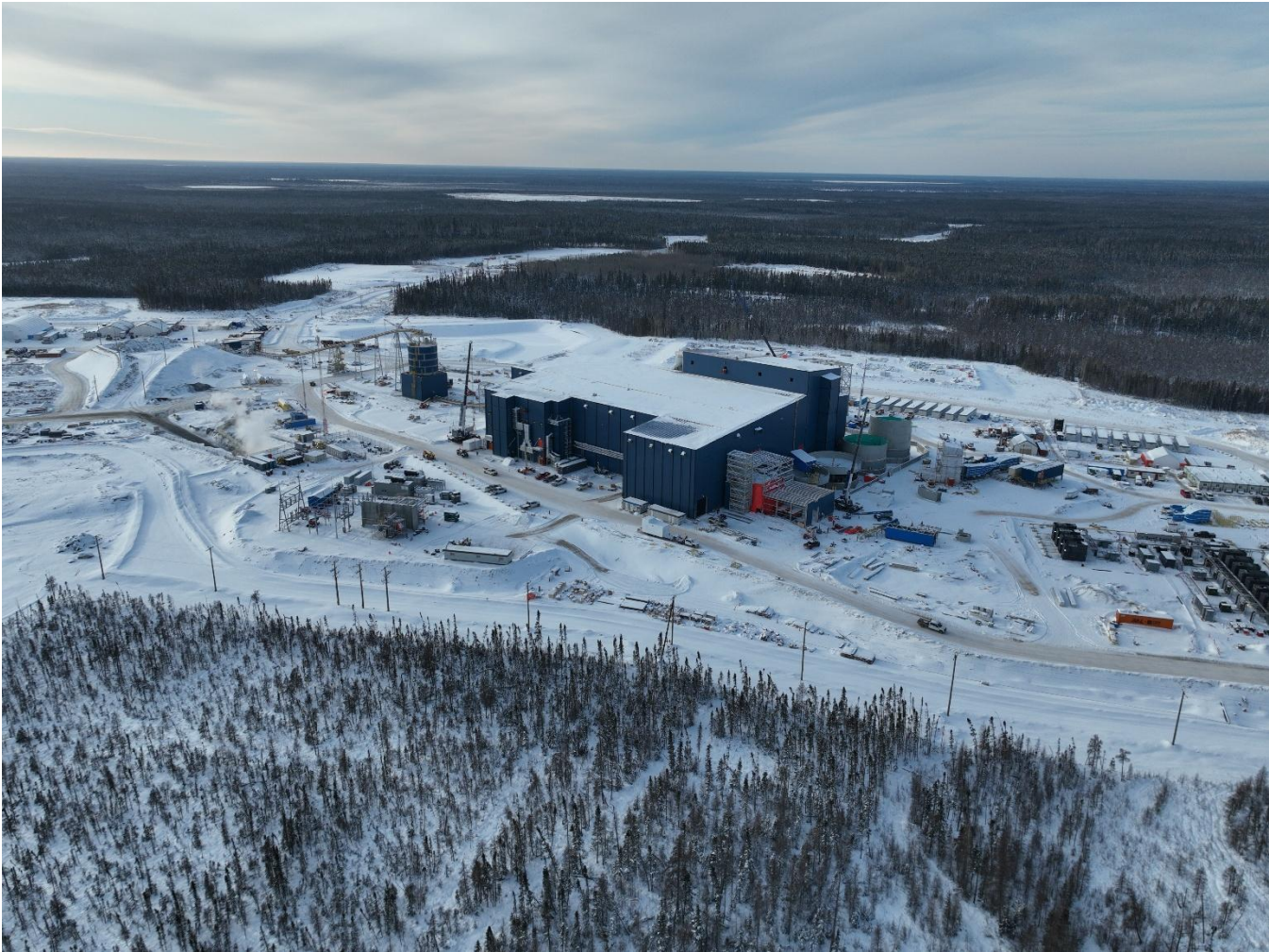
Site Layout – Looking West (Middle of December 2025)
