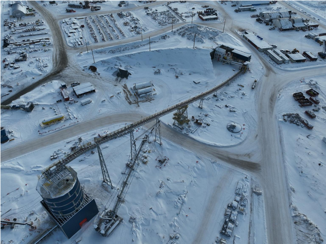
Primary Crusher and Conveyor Assembly (Middle of December 2025)
