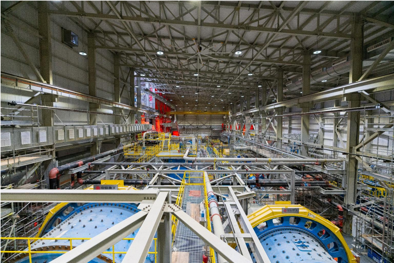
Process Plant Comminution Circuit (Middle of December 2025)
