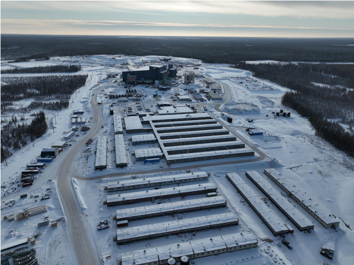
Site Layout – Looking South (Middle of December 2025)
