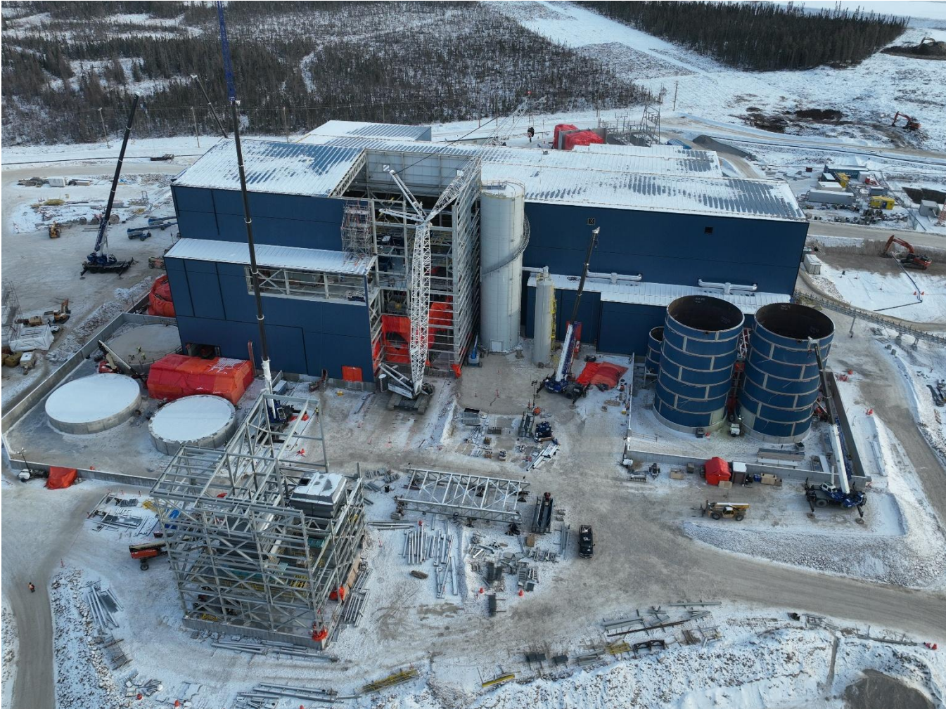
Process Plant – Looking East
