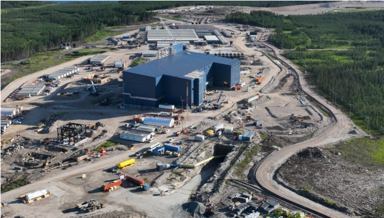
Site Layout – Looking North
