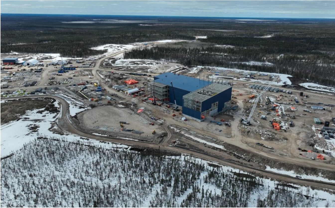
Site Layout – Looking West
