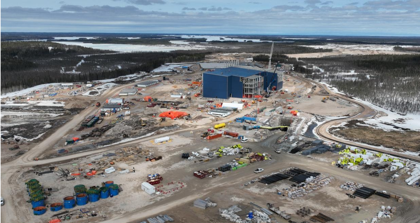
Site Layout – Looking North
