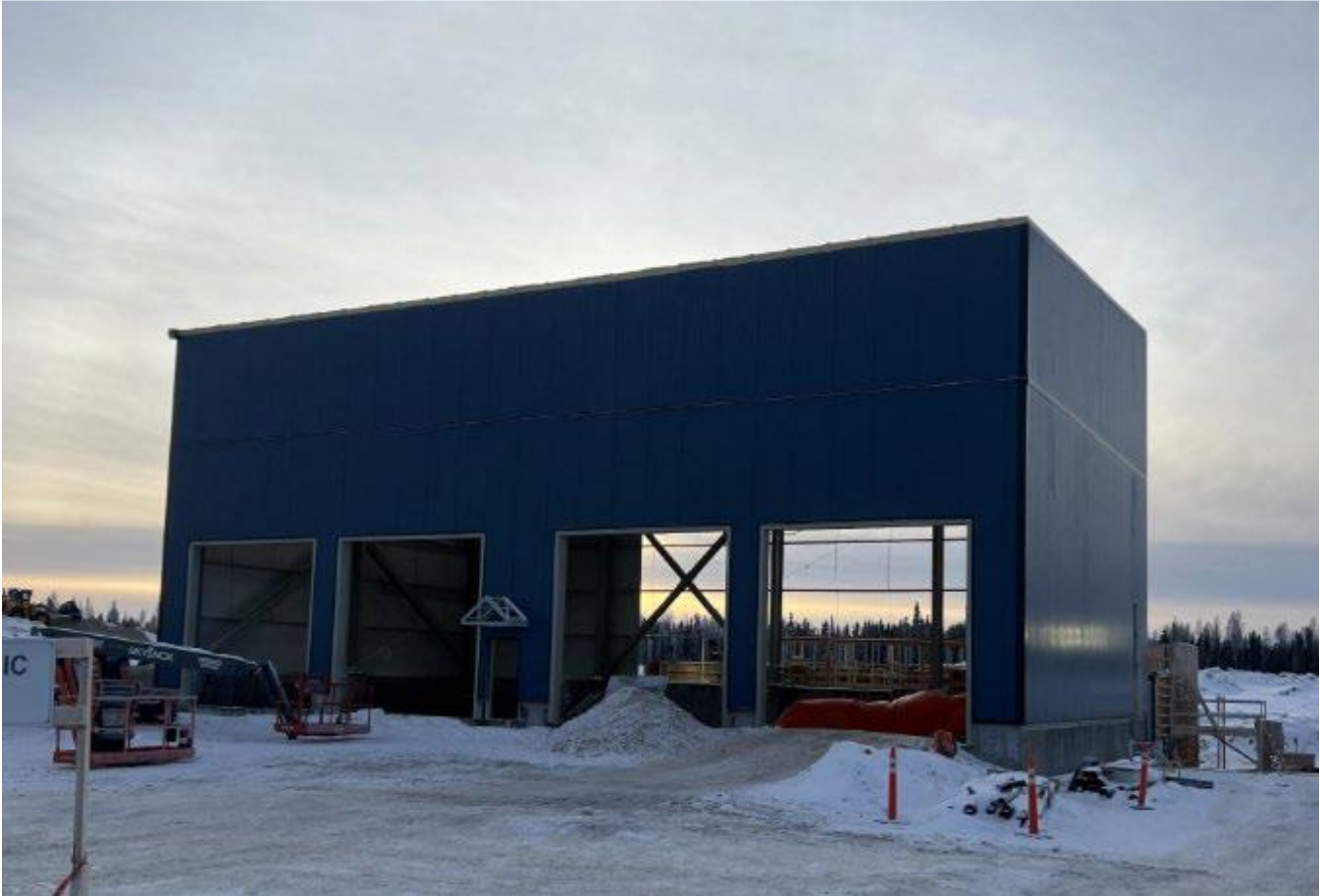
Surface Maintenance Shop with 3 x heavy equipment bays and BEV battery maintenance bay
