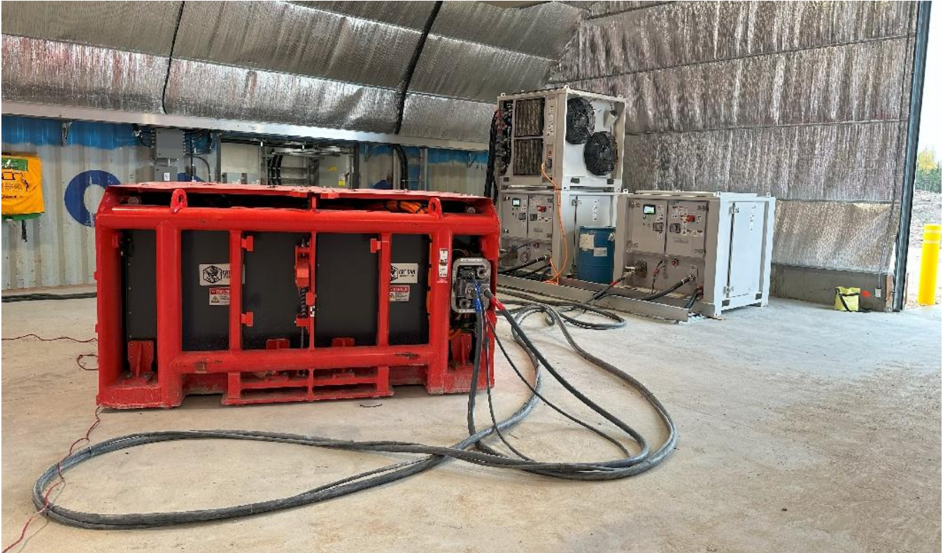
Battery Charging Station on Surface
