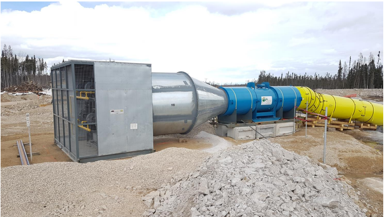
Figure 2 – Mine Air Heater with Fan
