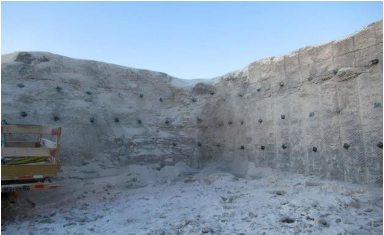
Figure 2 – Ground Support Installation in the Boxcut
