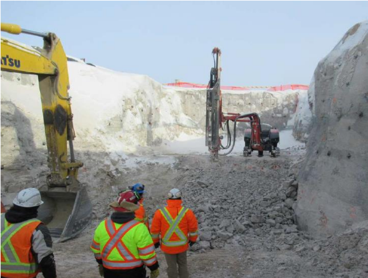
Figure 3 – Ongoing Drilling in Boxcut
